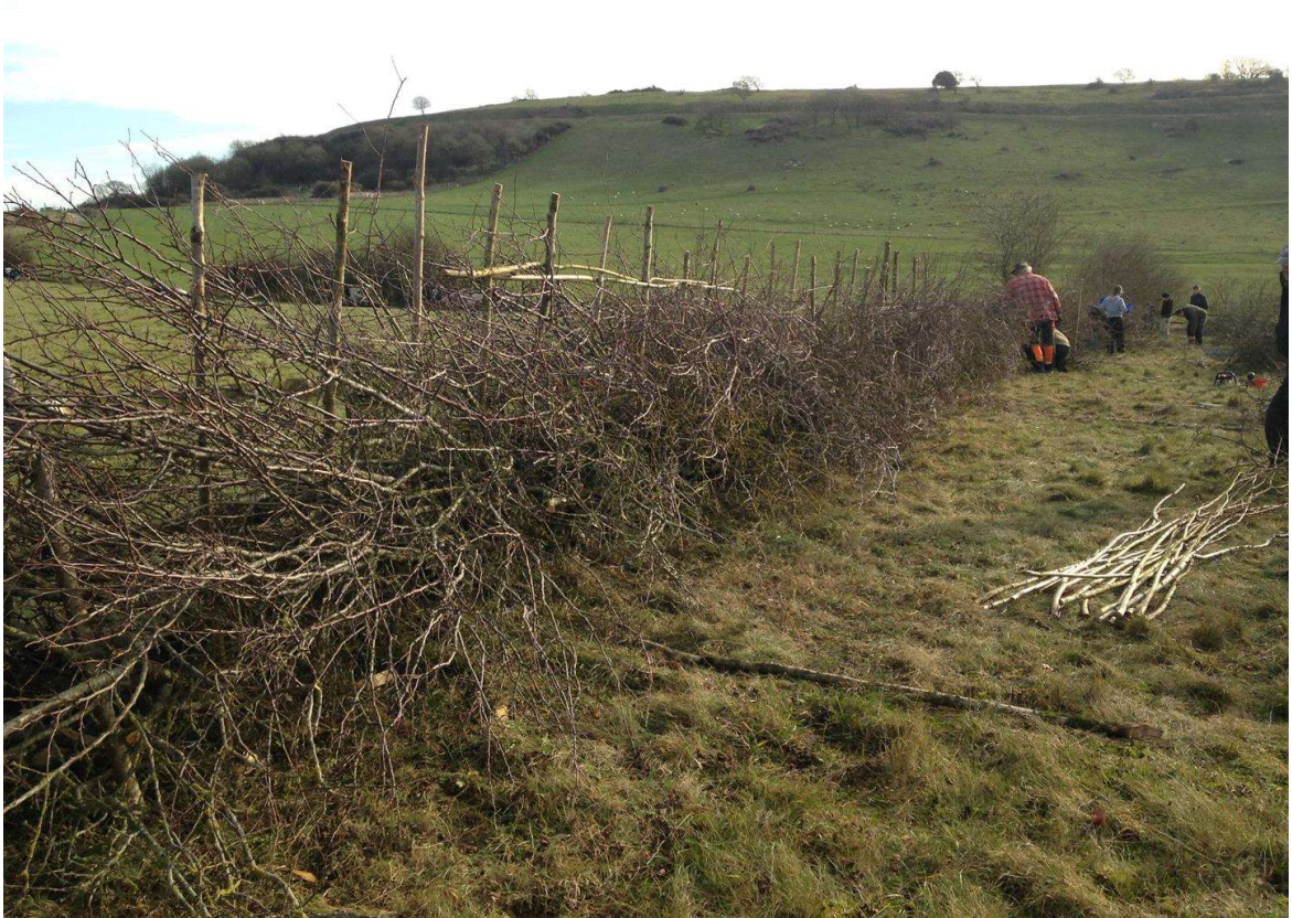
Fig 12: Once all pleachers are layed, stakes (approx. 5-6' x 2") are driven through at intervals of approximately 1' 6" apart (closed fist to elbow is a good measure) down the centre line of the hedge, helping to support the structure. Then binders (approx. 10-5' x 1.5") are woven alternately around the stakes (see Picture 8). Stakes and binders here are both hazel.
